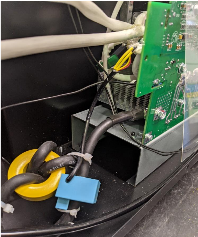
Figure 1 - Hall device tied in tight position
