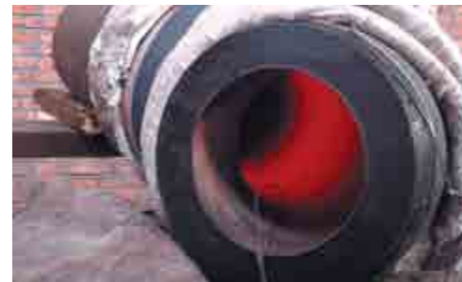
POST WELD HEAT TREATMENT ON P92 500MM DIAMETER X 90MM WALL
