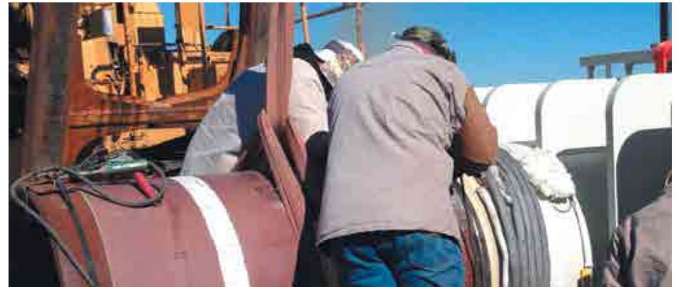
PRE-HEATING AND MAINTAINING INTER-PASS TEMPERATURE ON HEAVY WALL GAS PIPE
