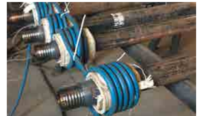
PRE AND POST WELD HEAT TREATMENT ON DRILL RODS
